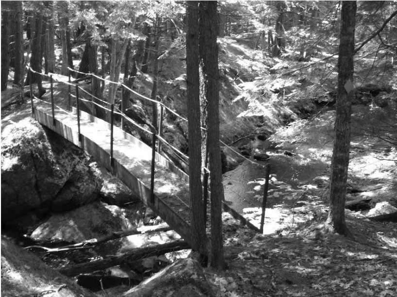
I-beam bridge over the Lane River on the Webb/Crowell Trail
